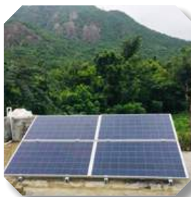
Solar water pumping system 1 HP (Odisha)
