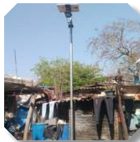
Integrated Solar Street Light 20W with PV rotation arrangement (Odisha)
