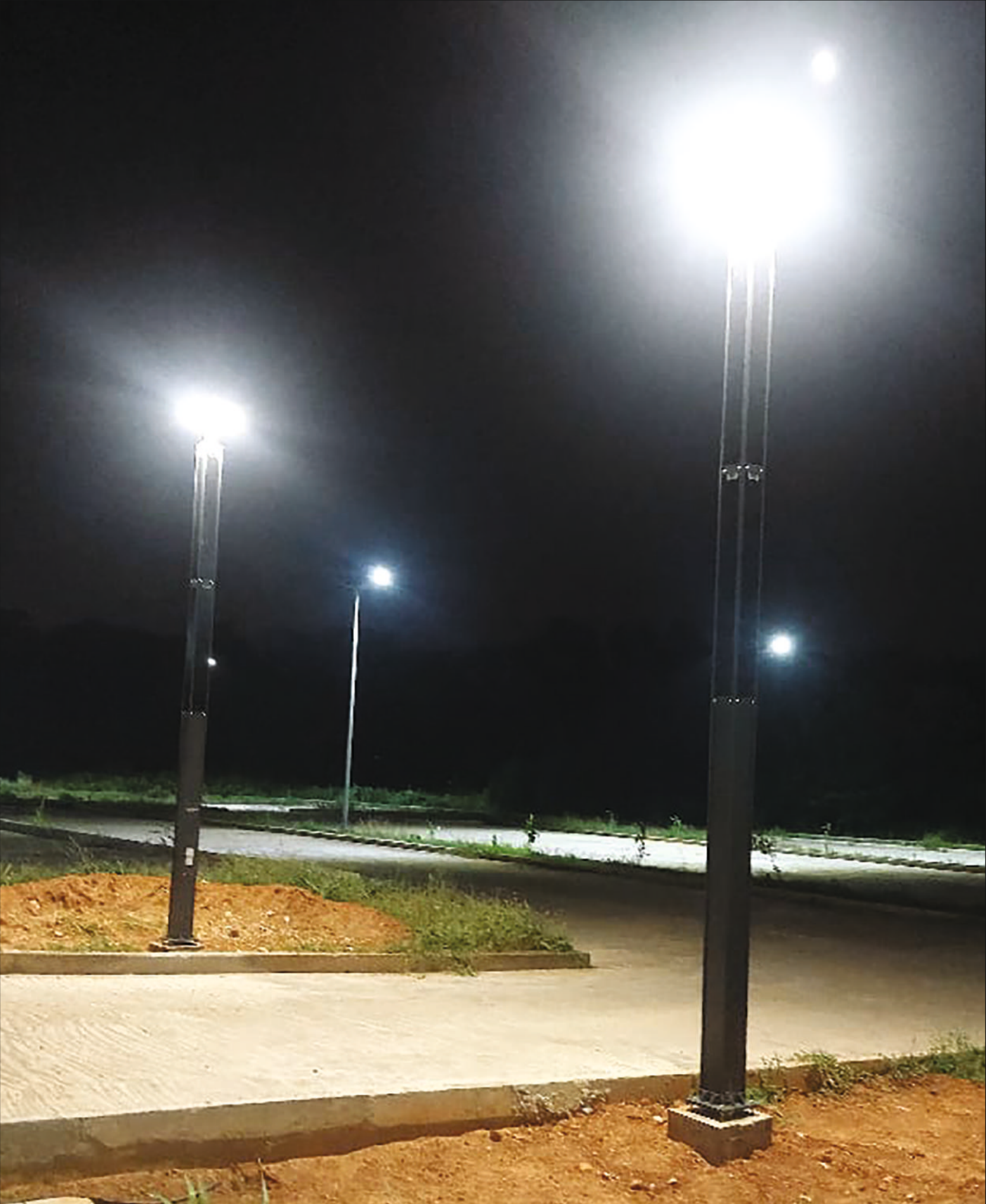
Actual site installation image of Solar Post Top Pole - Visakhapatnam
